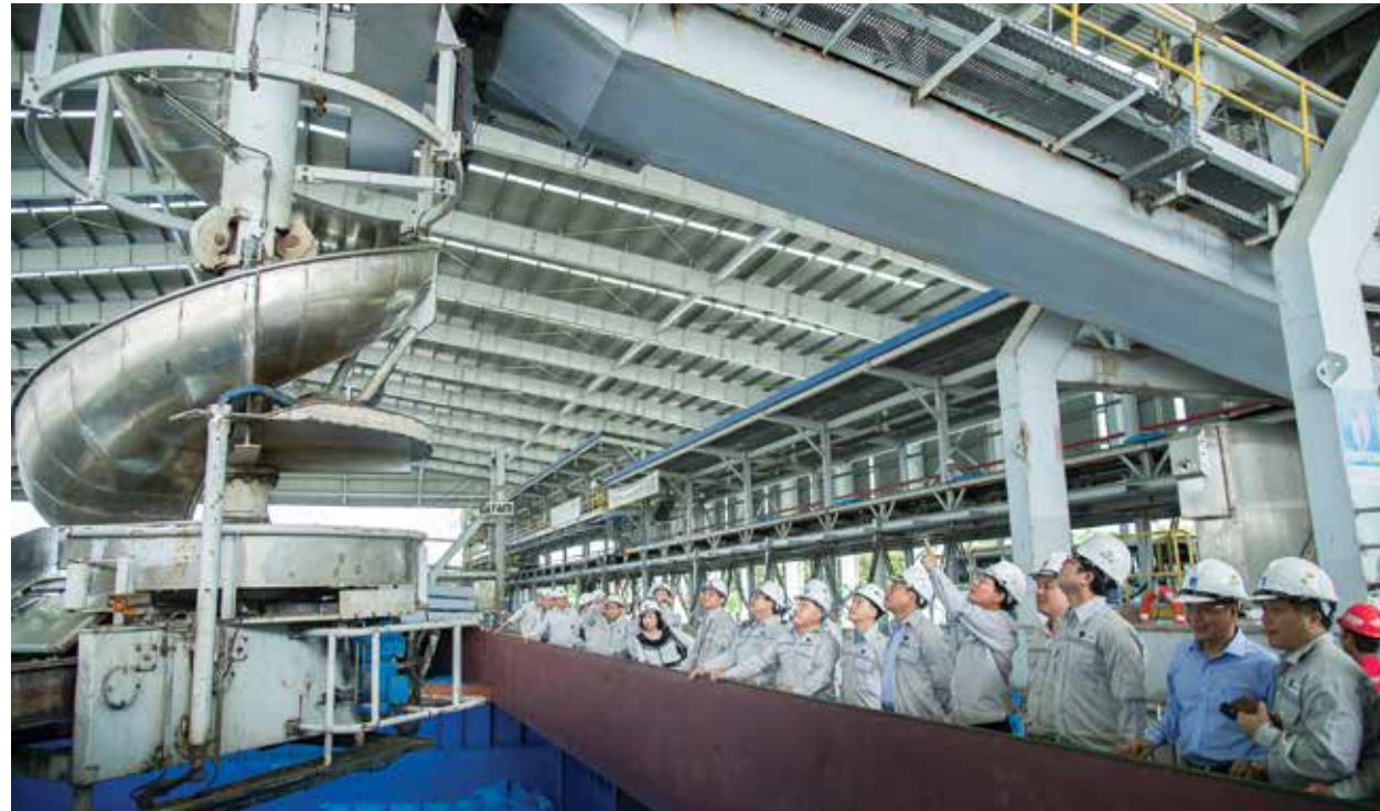
Automatic port system at Ca Mau Fertilizer Plant
